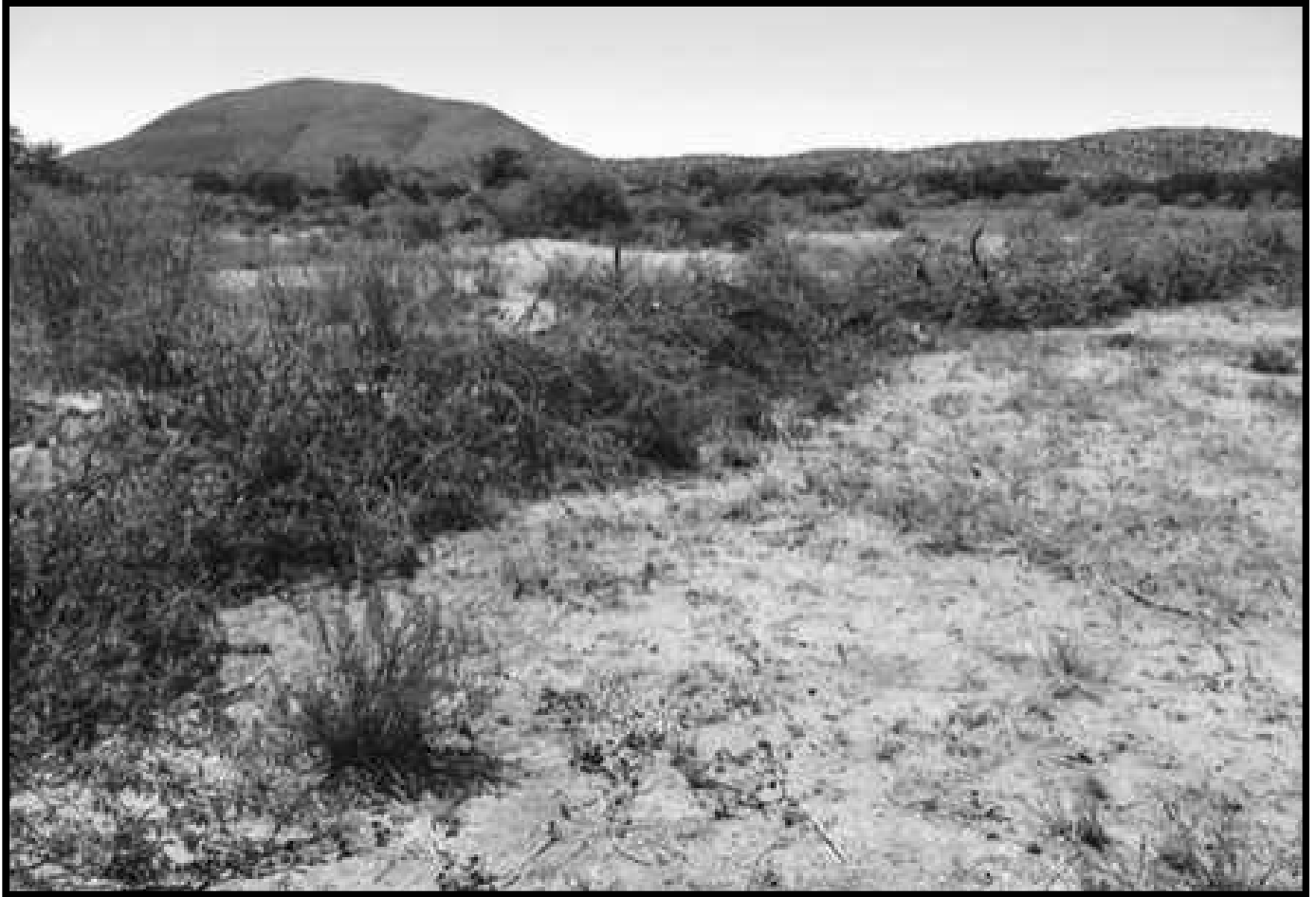
Figure 3. A filter of thorn bushes was tied down at a gully head.
